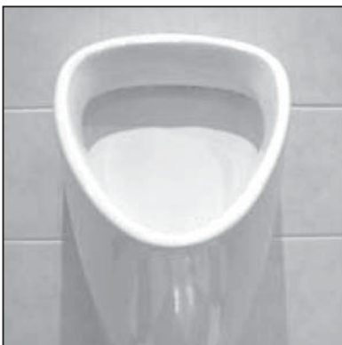
Put on the ceramics. Attention! Do not pen in the sensorcable! Open main water connection, turn on mains supply - ready to operate
