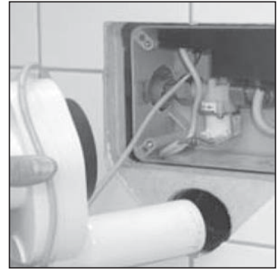
Insert sensorsiphon
