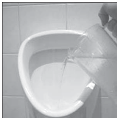
Check function: by pooring 1l water into urinal a flushing takes place.
